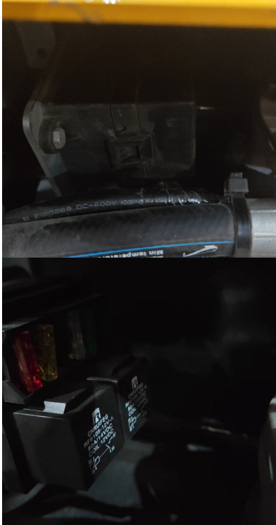
Fuse box, located under the battery
